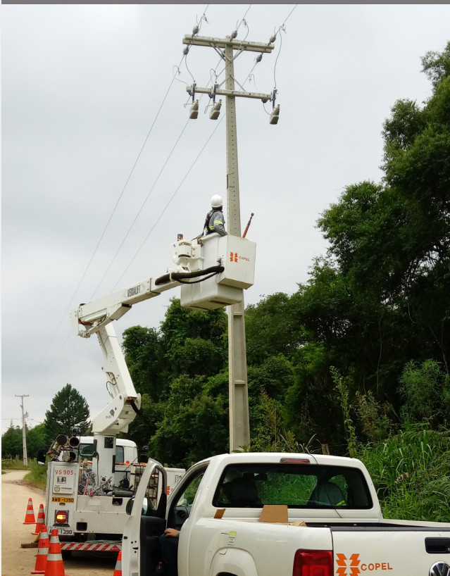
The COPEL team installs TripSaver II reclosers.
